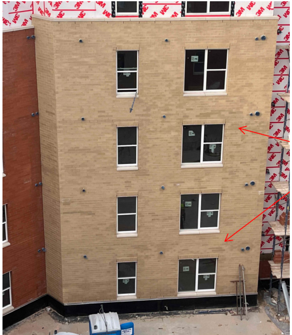
Photo 1: Reported color variation of brickwork in courtyard (mid-April)
